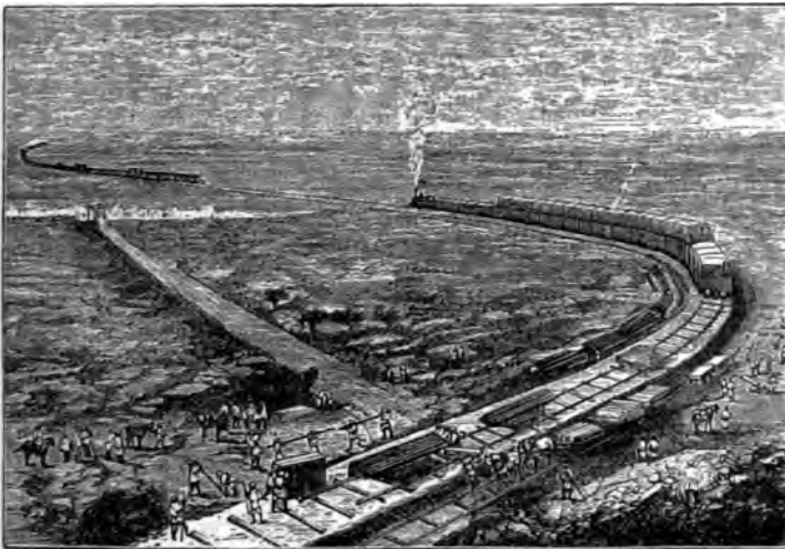
LAYING THE RAILS.
